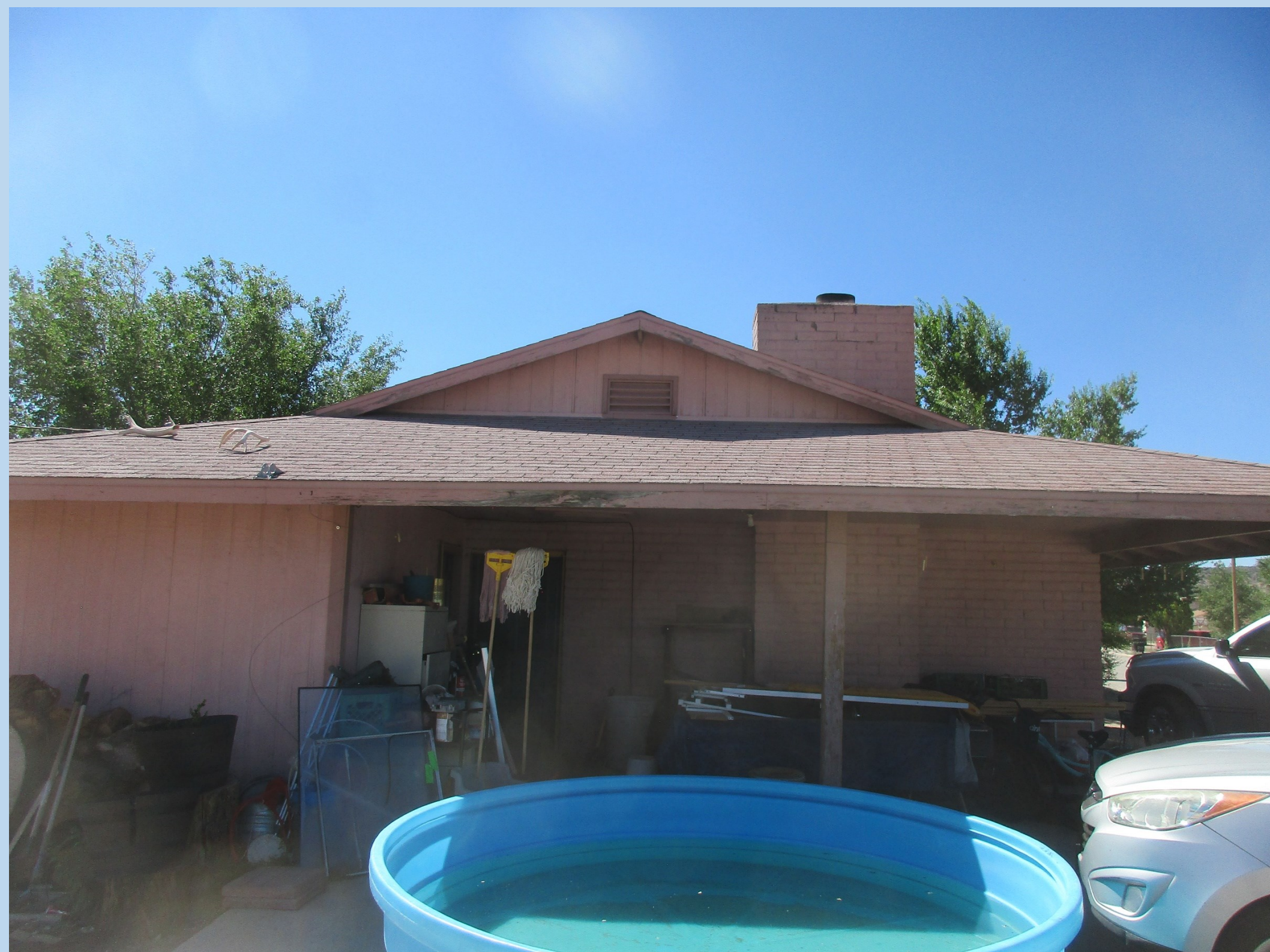
North view of Residence on Diamond Creek Road
