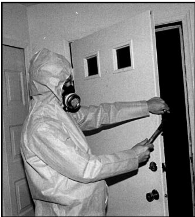
Figure 12.21 Use Punches To Identify the Location of Components Before Sending Them Offsite for Paint Removal.
