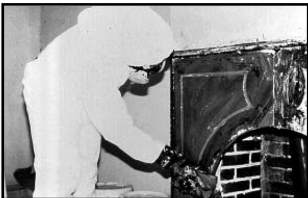
Figure 12.23b Neutralize Surfaces With a Glacial Acetic Acid Wash When Using Caustic Paint Removers.
