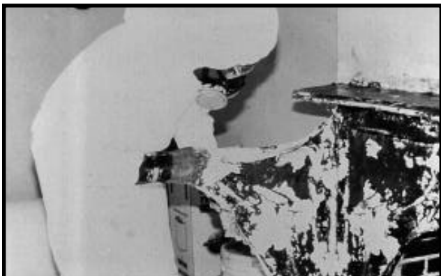
Figure 12.23a Neutralize Surfaces When Using Caustic Paint Removers.
