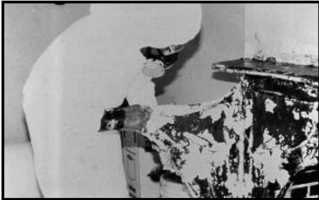
Figure 12.20 Proper Protective Gear, Including Gloves, Faceshield, Goggles, and Eyewash is Required When Working With Chemical Paint Removers.
