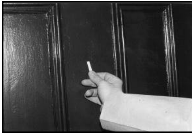
Figure 12.24 Use Litmus Paper on a Bare Stripped Surface Before Repainting.
