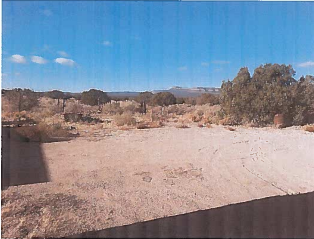
Green stake marking location of new Septic Tank to northwest of existing home.
