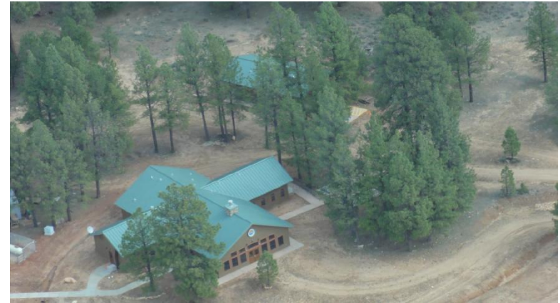
Aerial view of Bunk House & Laundry/Restroom building
